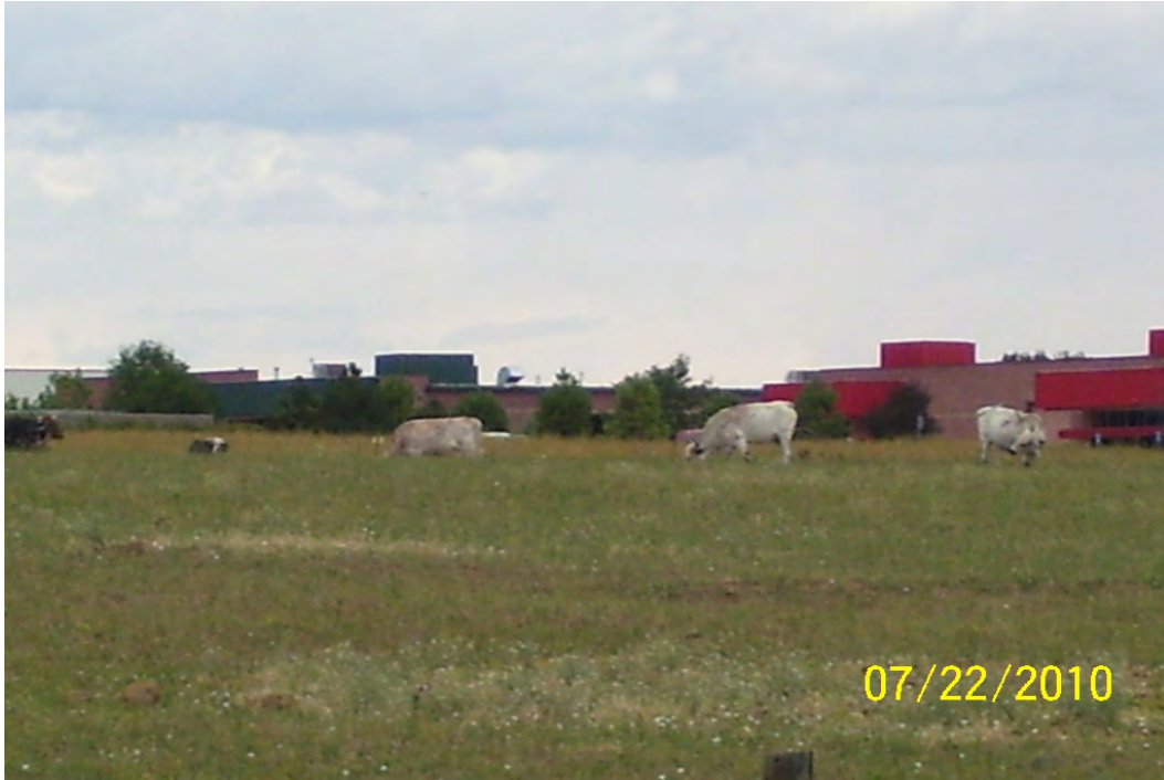
Other buildings on west side of parcels.
