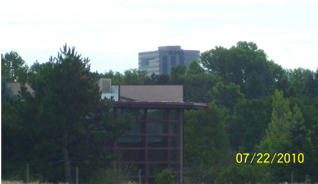
Residence on 13-001 with an office building in the background.
