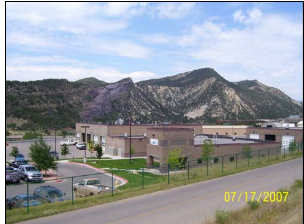
One of the capital projects La Plata County recently undertook included the building of a new road & bridge fleet maintenance shop.
